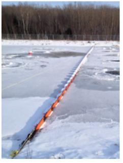
Baffles deployed in ice conditions
